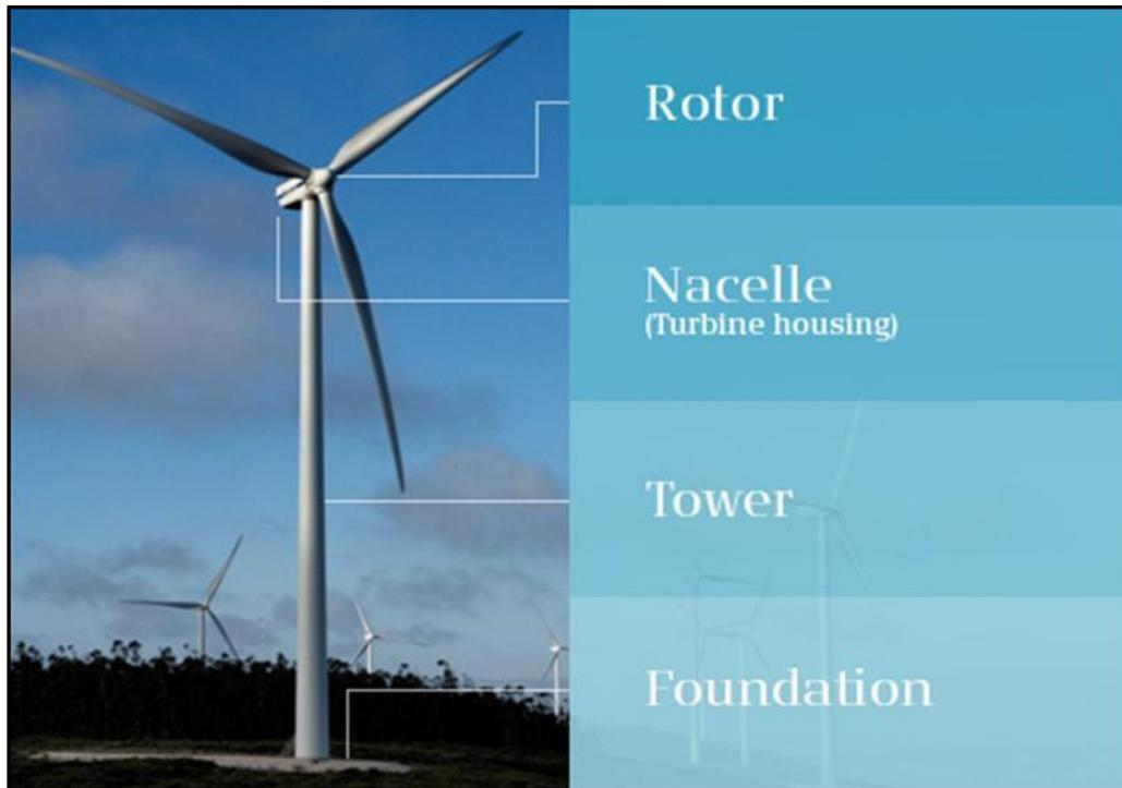
Plate 2-1 Wind turbine components
